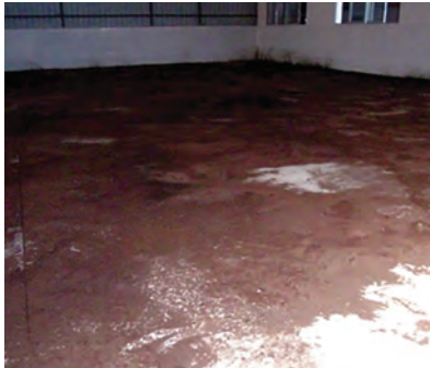
Black oxidized cement floor after preparation
