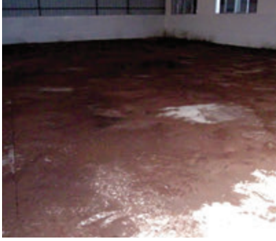
Black oxidized cement floor after preparation
